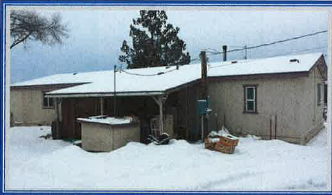
# 3 Rear (east) side of home.
