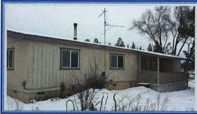
# 1 Front (west) side of home.
